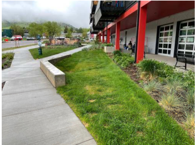
Photograph RPA-9. Grass buffer provides an opportunity for filtration and infiltration of roof runoff and disconnects impervious area of roof from inlet to storm drainage system.
