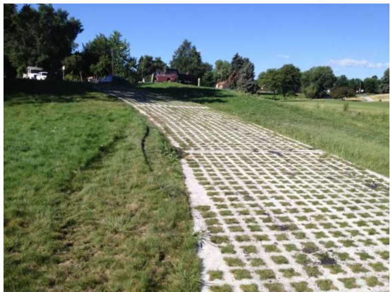
Photograph PPS-6. Reinforced grass pavement using concrete grid for maintenance access to a stormwater pond.
