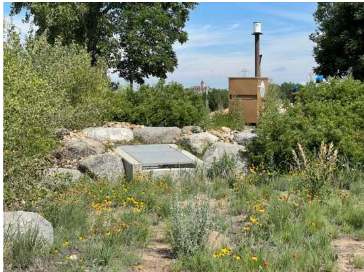
Photograph 4-17. Outlet for bioretention system at River Run Park. The WQCV is filtered through media and infiltrates or discharges to the outlet via an underdrain. The outlet is also designed for detention of larger events with a weir control (i.e., top of outlet box) and overflow spillway. The spillway is provided as a low spot above the outlet near the rain gage.
