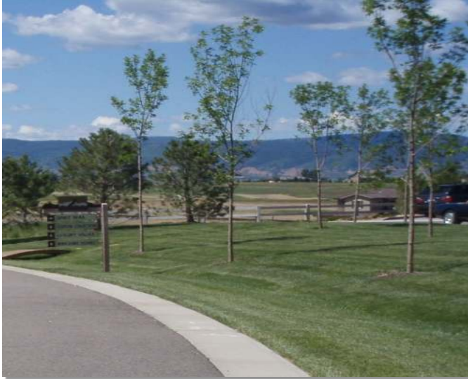
Photograph RPA-1. Grass buffers are often used in conjunction with grass swales as a treatment train. These pervious areas also help reduce heat island effects in urban areas. Photo: Muller Engineering.
