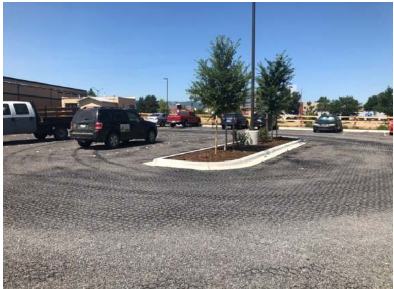
Photograph PPS-17. PGP parking area with markers to delineate parking spaces. Photo: True Grid
