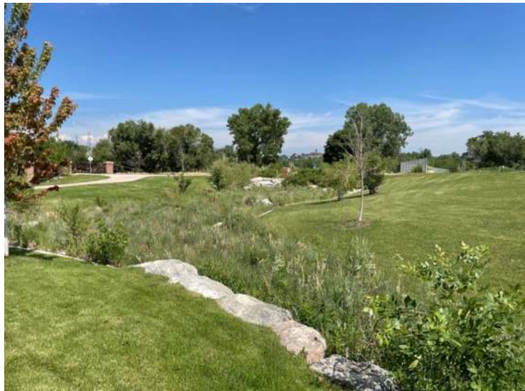
Photograph 4-2. Full spectrum bioretention system at River Run Park creates a natural area that complements the manicured upland turf grass areas and provides a transition from the urban environment to the river.
