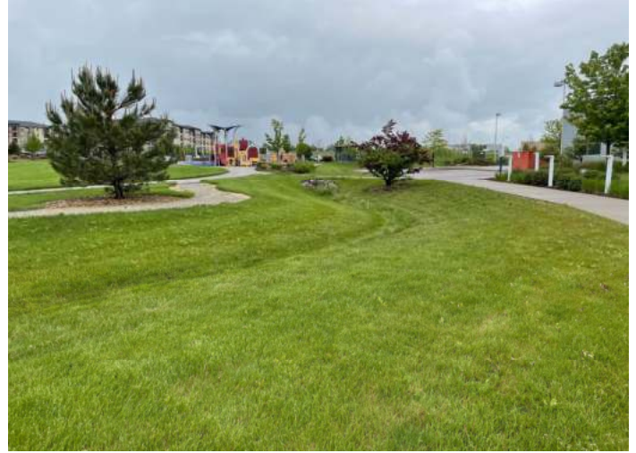
Photograph RPA-3. This grass swale provides treatment of runoff from a parking lot, portions of the building, and sidewalks at a healthcare facility. Photo: WWE.
