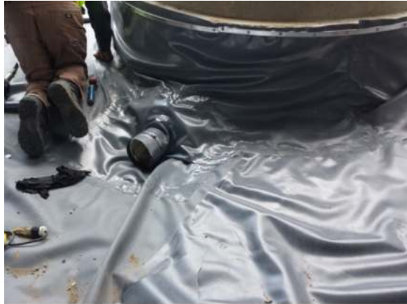
Photograph PPS-19. Underdrain penetration of geomembrane with boot. Photo: Creative Civil.
