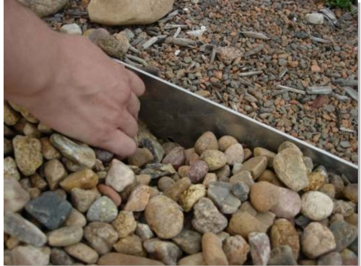
Photograph GR-4. The metal edging has perforations near the bottom to allow flow into the drain.
