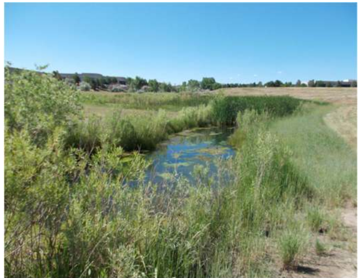
Photograph RP/CWP-2. Constructed wetland pond with diverse vegetation provides sedimentation, filtering and biological treatment.
