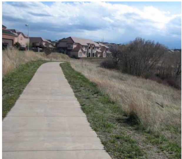
Photograph RPA-4. Grass buffers can be used to manage runoff from parking lots, multi-use paths, roadways, or roof areas, provided the flow is distributed in a uniform manner over the width of the buffer. Native grasses provide a more natural appearance. Photo: WWE.
