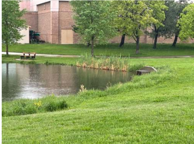
Photograph RP/CWP-7. This pond outlet structure is accessible and functional while not interfering with the overall pond aesthetic.
