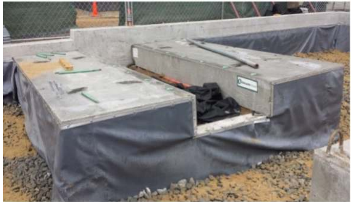
Photograph PPS-12. Tree planter vault for PICP installation. Photo: Creative Civil.
