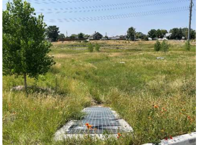
Photograph EDB-1. This EDB illustrates the use of a soft, meandering low flow channel and varied bottom grading with vegetation selected for the associated hydrologic conditions.
