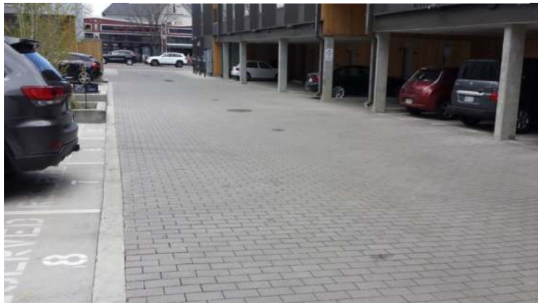
Photograph PPS-2. PICP in alley treats runoff from roof drains and adjacent parking spaces. A surface overflow path to the street provides drainage if the system is clogged or overwhelmed by runoff.
