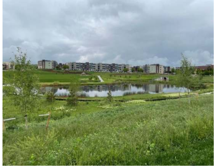
Photograph RP/CWP-1. Retention ponds and constructed wetland ponds treat stormwater through sedimentation and biological processes including uptake.
