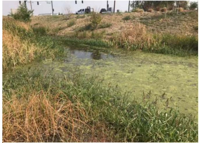
Photograph RP/CWP-6. Exceeding the minimum requirements for the permanent pool volume and depth can help to mitigate excessive growth of algae. Source control measures in the watershed that reduce nutrient loading may also be necessary.
