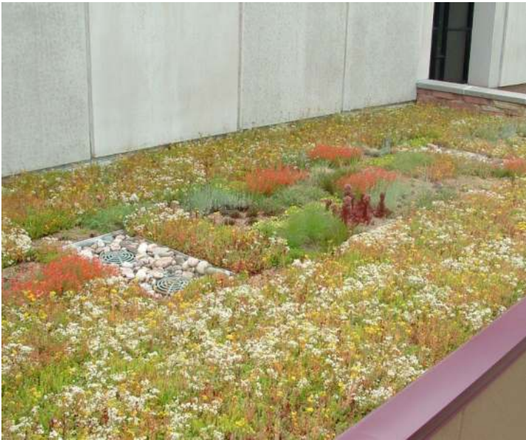
Photograph GR-1. Extensive Green Roof. Photo: Jennifer Boussetot.
