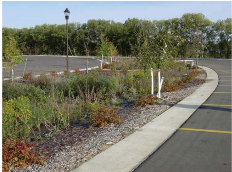
Photograph 4-9. Concrete edge acts as level spreader, distributing flow from parking lot as sheet flow to SCM.
