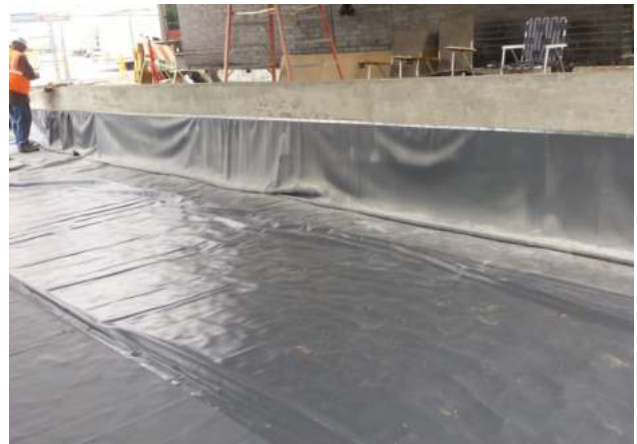
Photograph PPS-10. Geomembrane attached to concrete perimeter barrier. Photo: Creative Civil.
