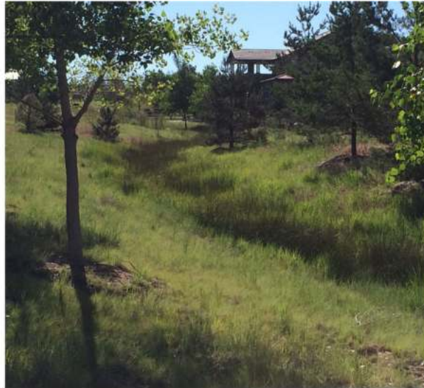
Photograph RPA-6. Dense vegetation in this 5% sloping swale provides the roughness to resist erosion and slow, filter, and infiltrate runoff.
