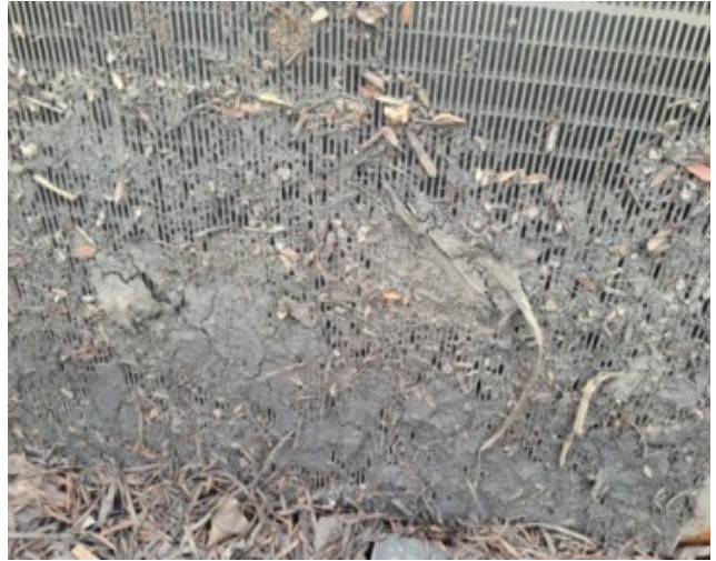
Photograph EDB-5. Well screen is intended to protect small orifices from clogging; however, the fine screen is itself subject to clogging and requires frequent inspection and maintenance to keep clear.
