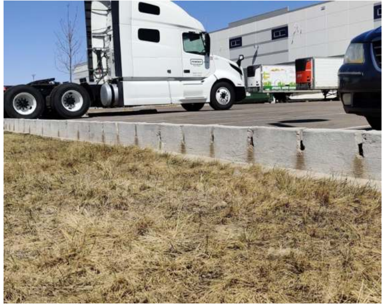
Photograph 4-8. Typical slotted curb showing drop from slot to adjacent pervious area to allow for growth of vegetation and sediment accumulation. This area provides for mowing and maintenance access to keep positive drainage from the parking lot to the RPA.
