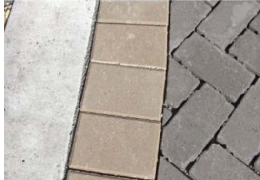
Photograph PPS-15. The very small cut paver shown in this photo could have been eliminated by rotating the paver above it 90 degrees.
