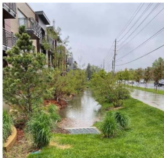
Photograph BR-2. Bioretention system treating urban stormwater during runoff event. Photo: Wright Water Engineers.
