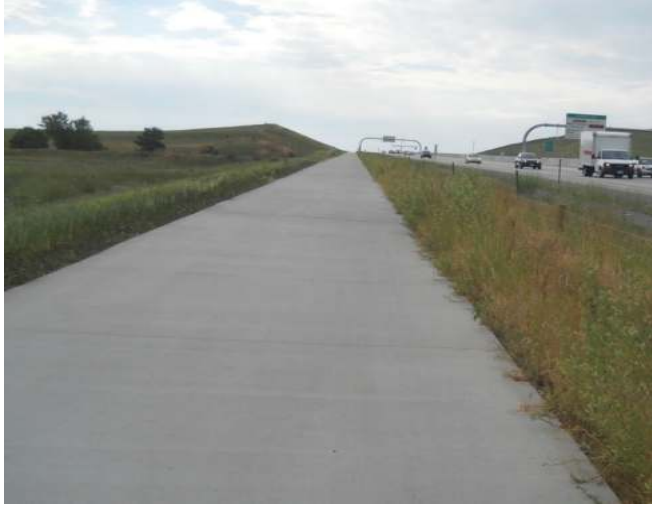
Photograph RPA-2. RPAs including grass buffers and swales treat runoff by filtering and infiltration. For treatment to be effective, RPAs must receive runoff as sheet flow. Photo: WWE.
