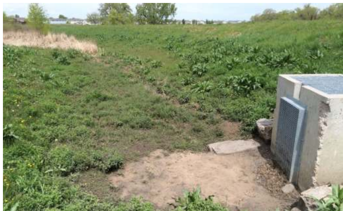
Photograph EDB-7. This EDB was originally constructed without a micropool and was retrofitted with a sand filter with underdrain to reduce the potential for clogging the outlet and water backing up in the basin.
