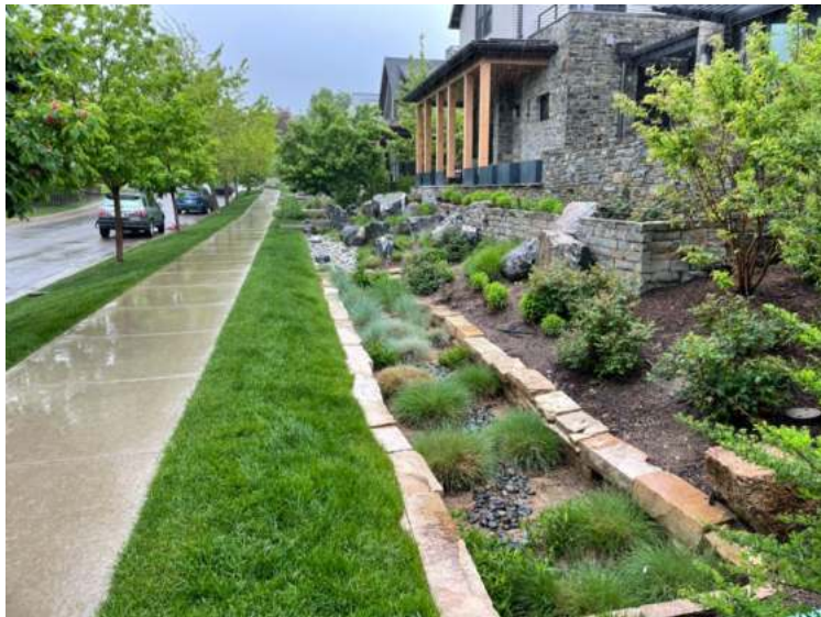
Photograph 4-3. Choice of materials for bioretention system is compatible with landscaping and aesthetics of neighborhood.
