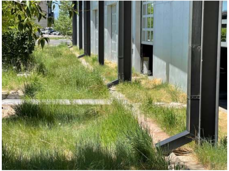
Photograph 4-14. Disconnected downspouts discharge to grass swale to dissipate concentrated flows and allow for infiltration and filtration. Vegetation provides energy dissipation.
