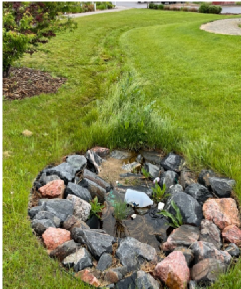
Photograph 4-15. Inlet to swale has small riprap forebay to collect trash. Riprap and dense vegetation in swale dissipate energy. However, sediment will be difficult to remove from the riprap.
