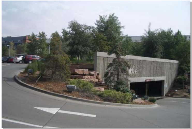
Photograph GR-3. Intensive green roof over parking garage is readily accessible for maintenance.
