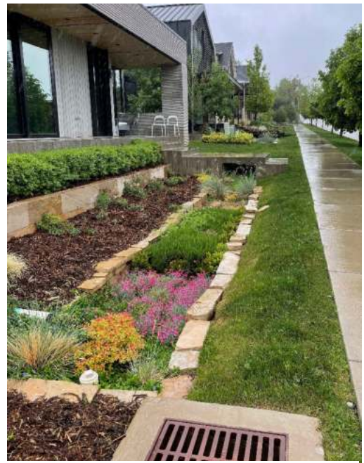
Photograph BR-1. This bioretention area treats runoff from the roof and lot, while serving as an aesthetically pleasing landscape feature. Photo: Wright Water Engineers.
