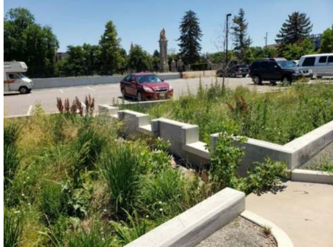
Photograph BR-3. Terraced bioretention SCM in recreation center parking lot. Photo: MHFD.
