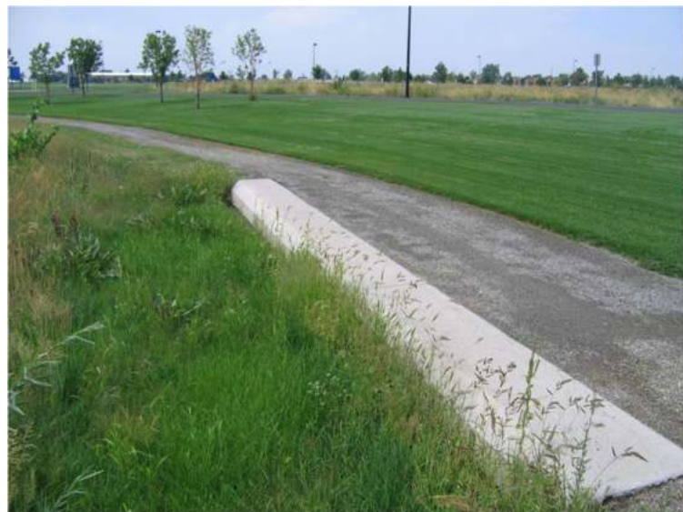
Photograph 4-12. Aurora Sports Park Level Spreader. This level spreader carries concentrated flows into a slotted pipe encased in concrete to distribute flows evenly to the RPA shown left in the photo. Photo: Wenk.
