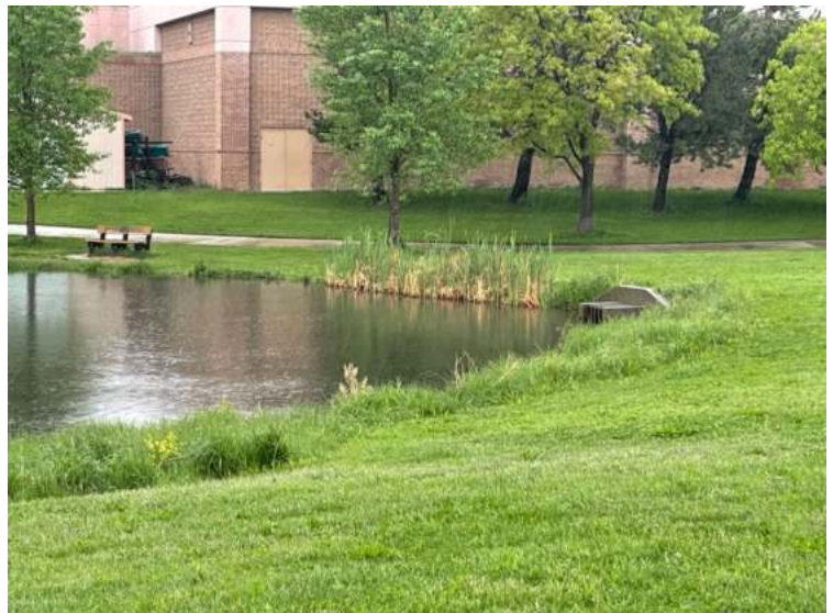
Photograph 4-19. Retention pond outlet structure blends with the bank and is easily accessible for maintenance.
