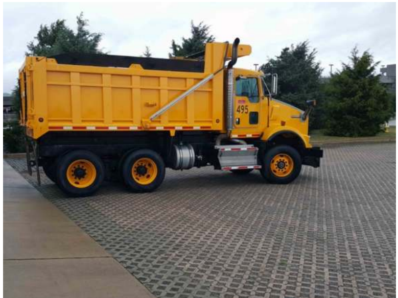
Photograph PPS-4. CGP installation allows for infiltration into subsurface via permeable infill material. Photo: True Grid.
