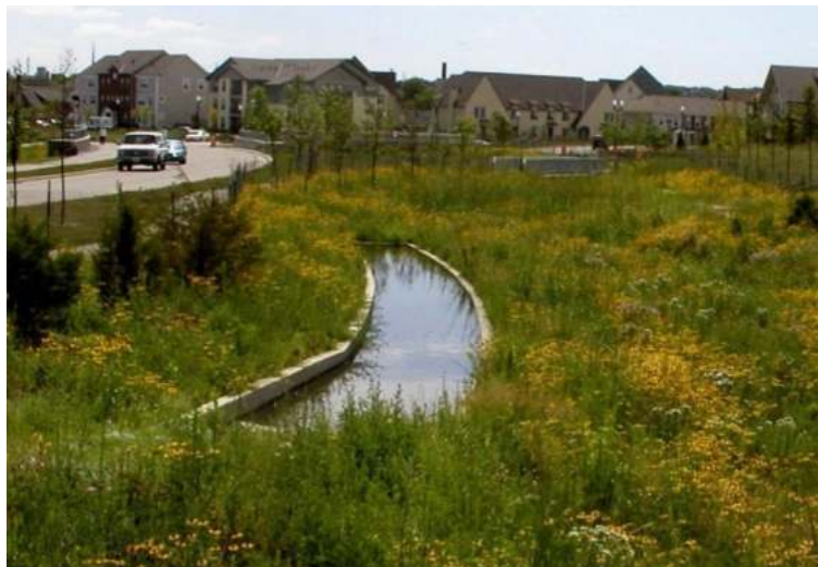
Photograph 4-10. This level spreader distributes concentrated piped inflows from the road to the buffer to the right in the photograph. The concrete sill to the left is the level spreader, and the flat shallow channel with water is the blind swale. Photo: Wenk.
