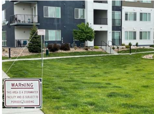
Photograph RPA-7. RPA in multi-family residential neighborhood. Sign warns of periodic flooding which helps establish expectations for periodic temporary ponding, while providing a safety warning. Photo: WWE.
