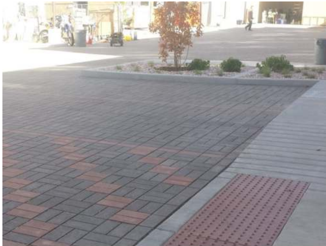
Photograph PPS-8. PICP with striped ADA parking and tree planter. Photo: Creative Civil.
