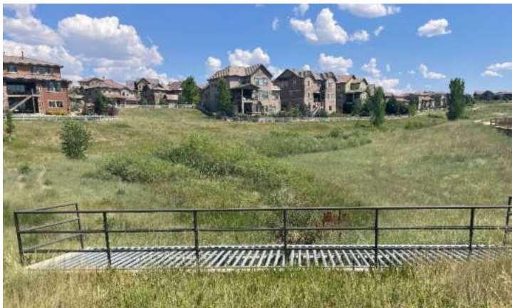
Photograph EDB-2. This EDB depicts a meandering low flow channel with adjacent benches that remain drier to allow equipment access for maintenance.
