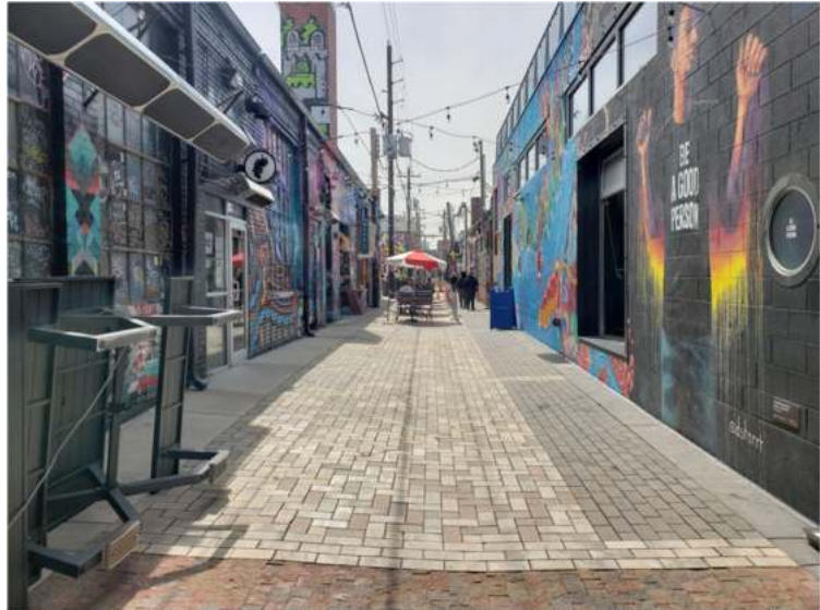
Photograph 4-1. Permeable pavement in an alleyway provides infiltration in a space-constrained environment and provides a multi-functional area valued for more than just stormwater treatment.
