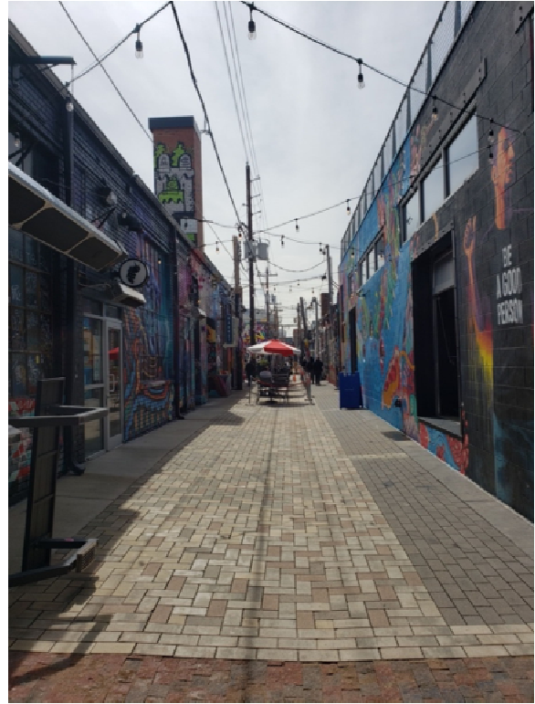
Photograph PPS-1. PICP in alley provides stormwater treatment in a retrofit setting while also providing outdoor seating and an attractive pedestrian area.
