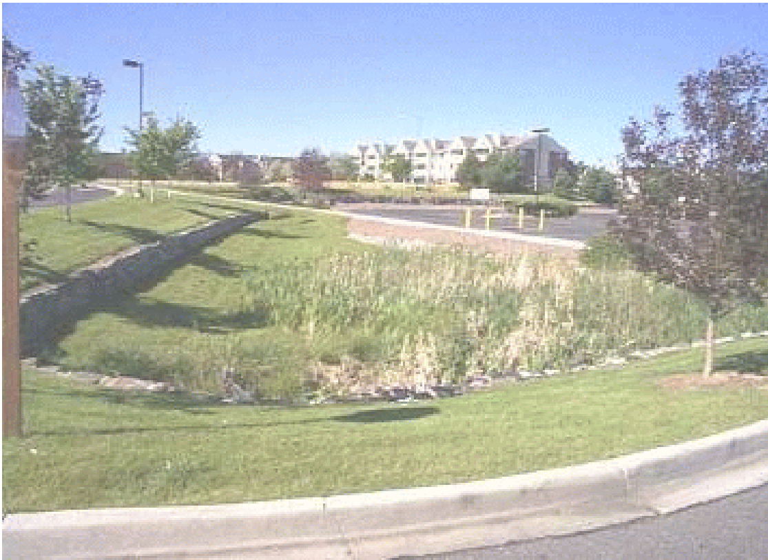
Figure 2-1 Typical Dry Pond (UDFCD, 1999)
