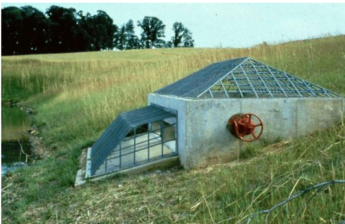
Figure 3-12 Typical Principal Spillway Outlet Structure
